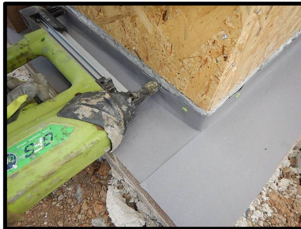
Apply TERM-seal Adhesive, TERM-seal™ Sealant Active or TERM-seal™ Multi-Purpose Active
