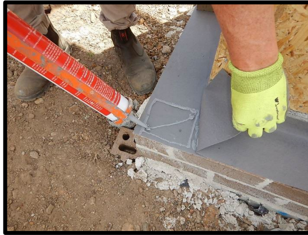
Apply TERM-seal Ura-Fen Adhesive, TERM-seal™ Sealant Active or TERM-seal™ Multi-Purpose Active to Perimeter Overlap
