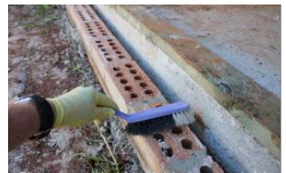
Clean excess dust from brick course and slab edge
