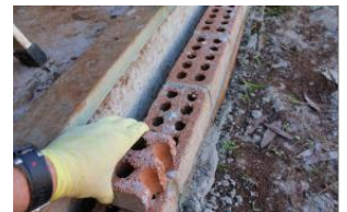
Clean surface of brick course and slab edge using spare brick to remove any excess mortar dags
