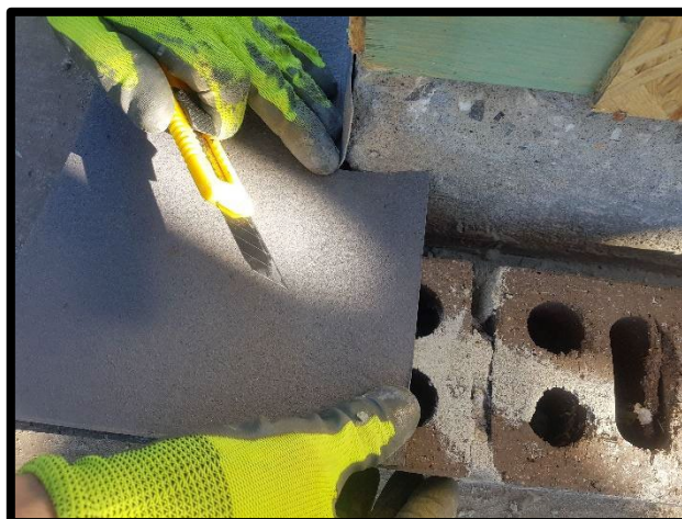
Created Flap placed on top of brick course
