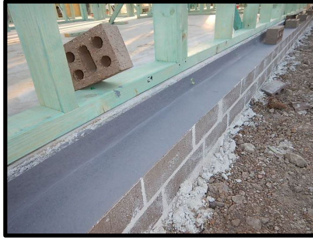
Figure 1 Side-Loading TERM-seal™ PRM Active Capping
