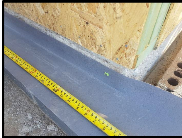
Correct Position of TERM-seal™ PRM Active Capping
