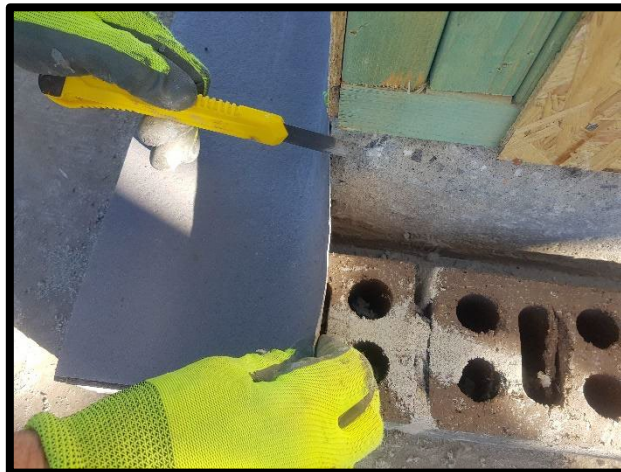
Vertical Cut Adjacent to The Slab Edge
