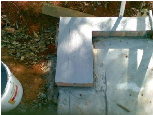
Infill garage where sealant is used in concrete joint
