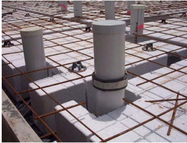
Fig.26 Void former fitted to (DWV) PVC pipe
