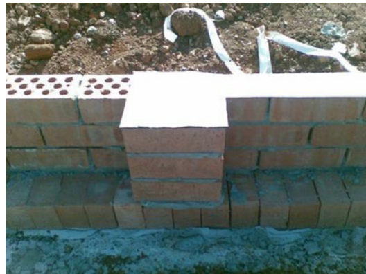
Bearer and joist, Engaged pier and wall
