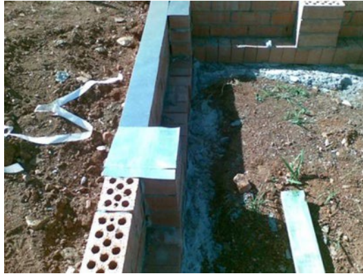
Engaged pier capping
