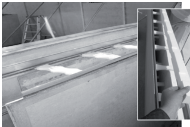
For increased speed of panel installation fix the panel joiners to the panel before erecting.
