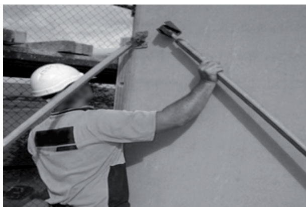
Secure brace foot plate to slab with Excalibur bolt and brace to panel with self-tapping screws into panel stud. Proceed to plumb panel in all directions utilizing the brace's push pull mechanisms and a level.
