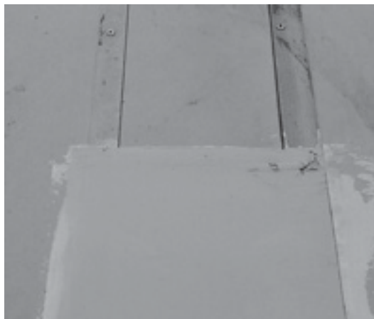
SETTING OF T-JUNCTION CLOSERS FIGURE 5.10
