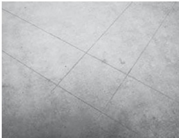
Set out the Tee Junction to surveyors pins
