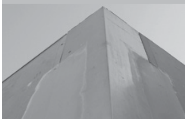
BASE COAT APPLIED TO CORNER CLOSER FIGURE 5.7
