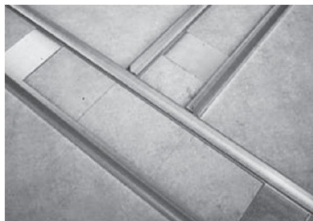
T-Junction Bottom Plate Set-out
