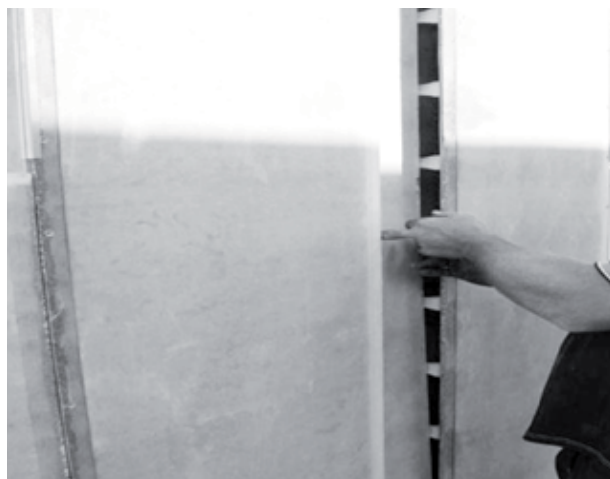
Place Tee Closure into position ready for closing off
