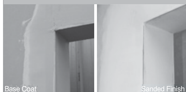
BASE COAT WINDOW / DOOR OPENING FIGURE 5.9
