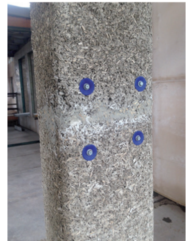
Plastic washer and long gal screw - on a narrow Hempcrete column
