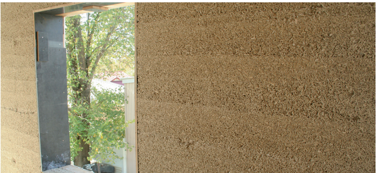
IMAGE CREDIT: D'Alo Constructions, VIC
