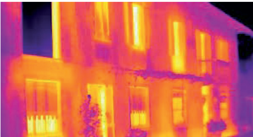
Thermographic image of a house
