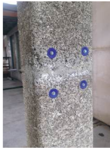
Plastic washer and long gal screw - on a narrow Hempcrete column
