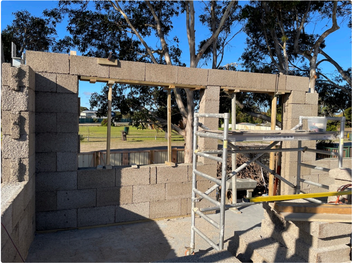
Above a picture of timber lintel block supports.
