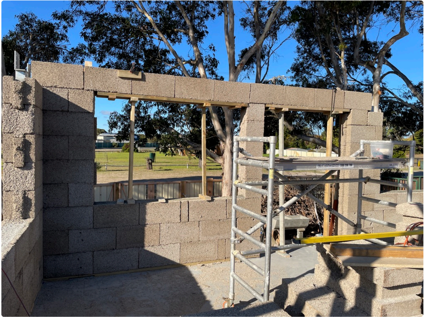
Timber lintel block supports.
