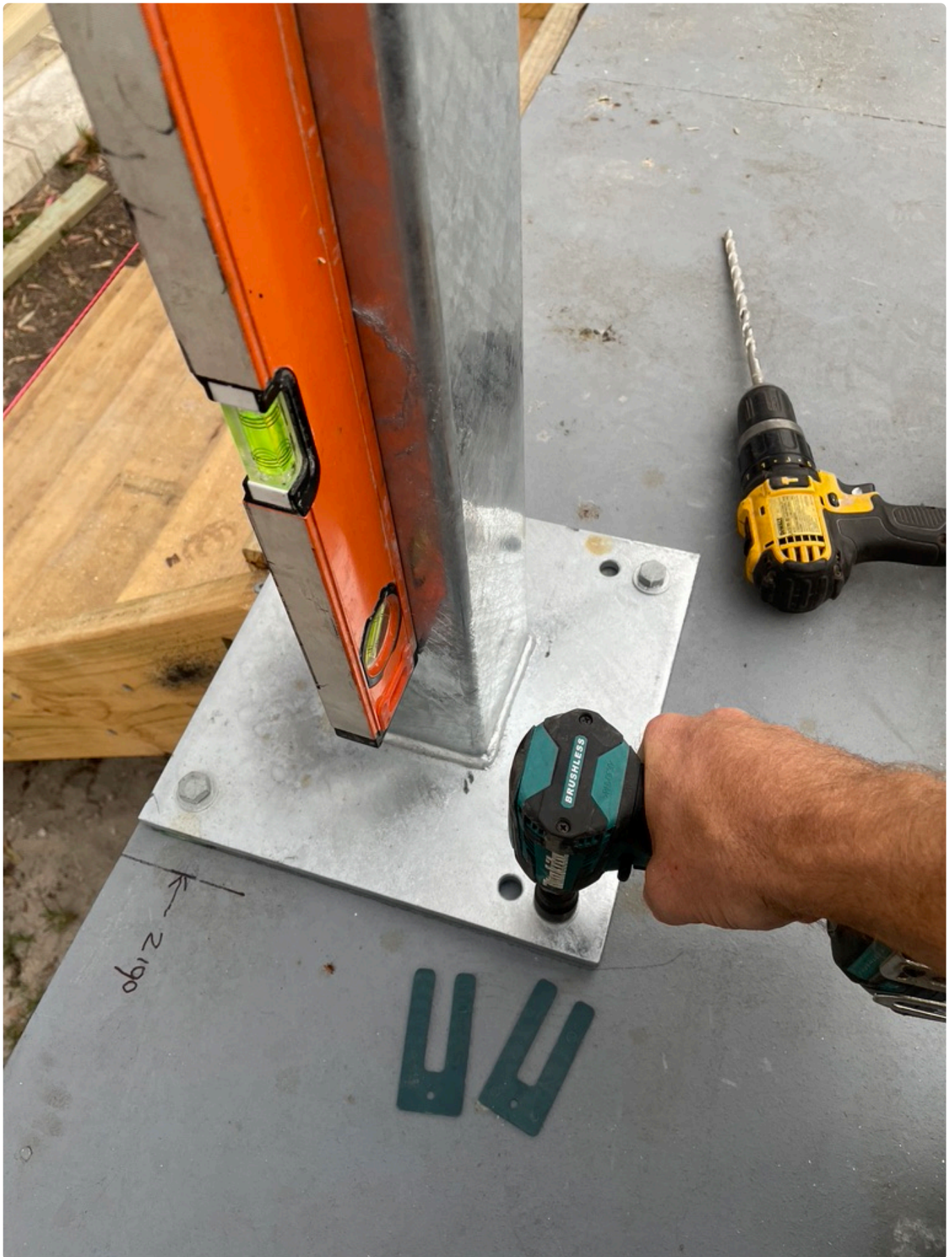
(the screws are connected to joists that are positioned under the floor)
