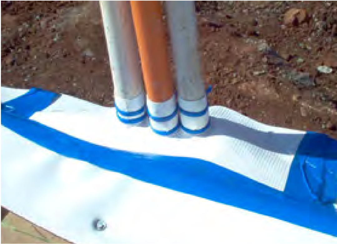
Above: Multiple penetrations in the perimeter cavity using HomeGuard® DPC
