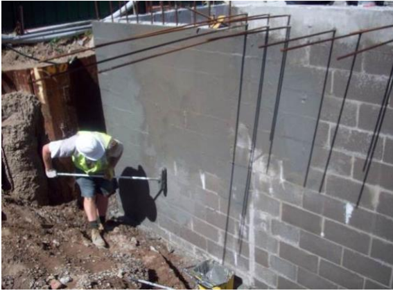
Figure 3 Ensure block work has been wet down with water before applying the first coat of NOVITHOR Cementitious Parge using a soft broom. (This will ensure product penetration and adhesion to block work.)
