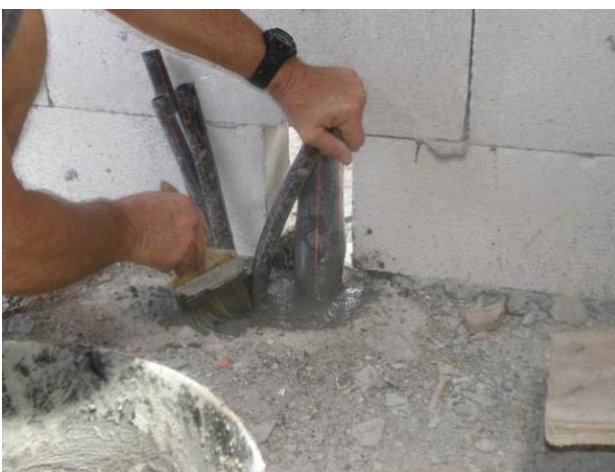
Figure 20B Apply NOVITHOR Cementitious Parge with soft bristled brush.
