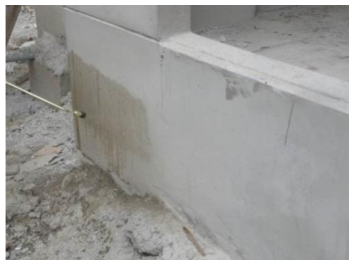
Figure 38 NOVITHOR Resin applied to rendered wall.
