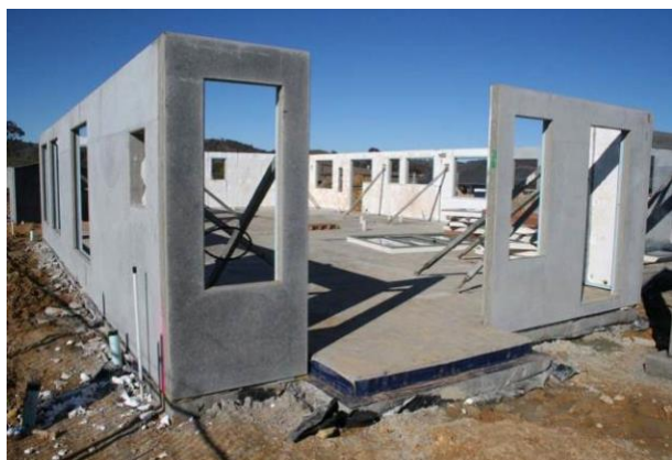
Figure 24 Tilt panel slab placed by builder.
