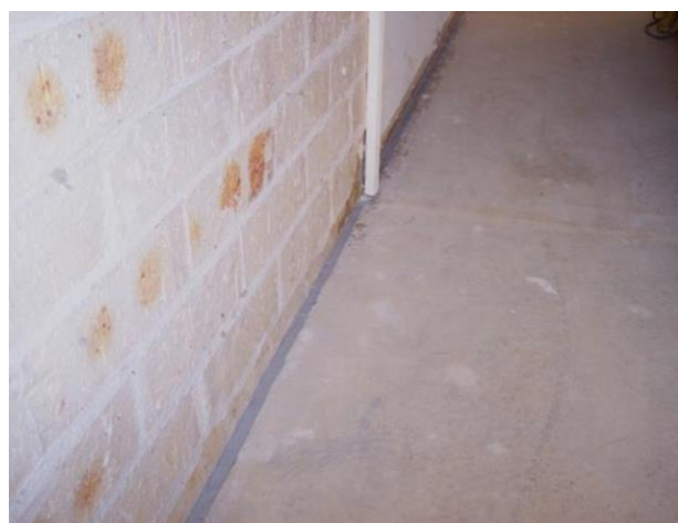
Figure 47 NOVITHOR Flexi-Gel between footing and garage floor in-fill slab.
