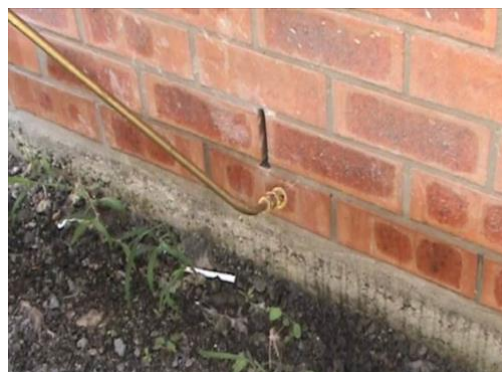
Figure 39 Applied to face bricks work. 1 st coat focus on mortar joints; 2 nd coat cover brick face to blend any runs.
