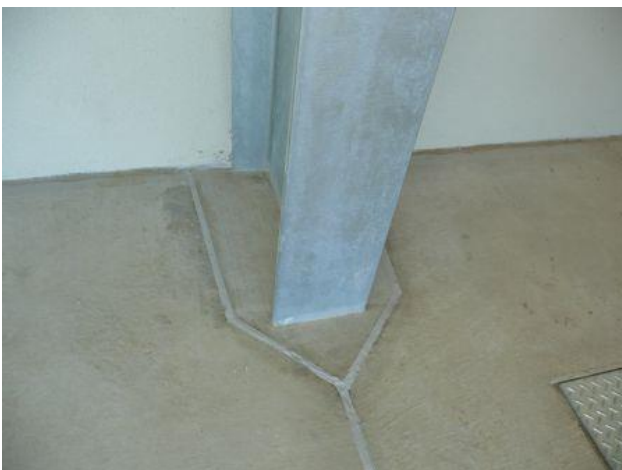
Figure 50 NOVITHOR Flexi-Gel around column.
