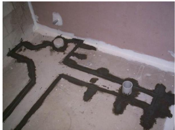
Figure 12 NOVITHOR Cementitious Parge over cold joint between old and new concrete and around pipe penetrations.
