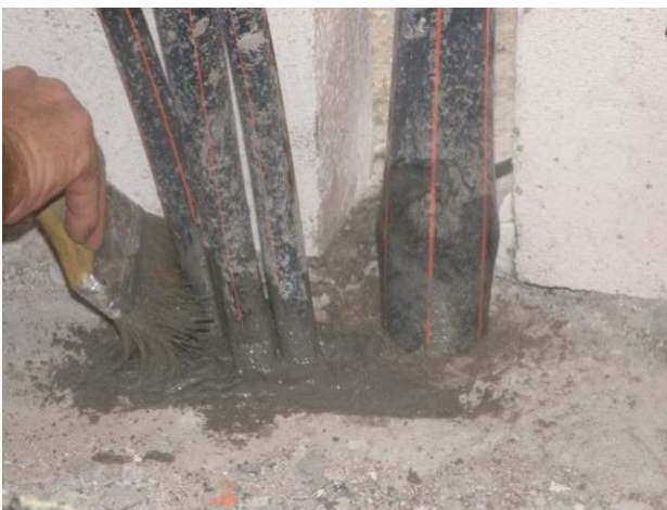
Figure 19 Apply NOVITHOR Cementitious Parge with soft bristled brush.
