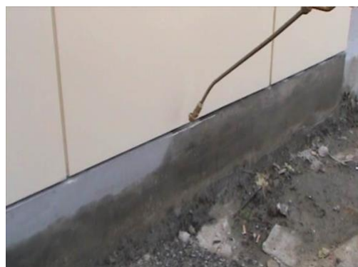
Figure 40 Resin being applied to rendered wall.
