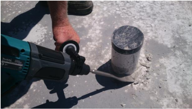
Figure 15 Using a rotary hammer drill with a flat chisel bit, chip out a recess in the slab approx. 5 mm deep.
