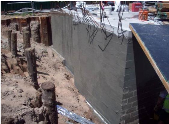
Figure 4 First coat is left to dry.
