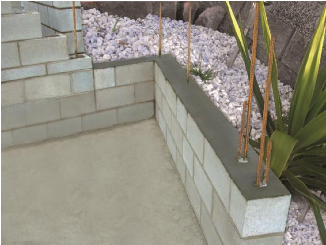
Figure 32 NOVITHOR Cementitious Parge capping RC block wall
