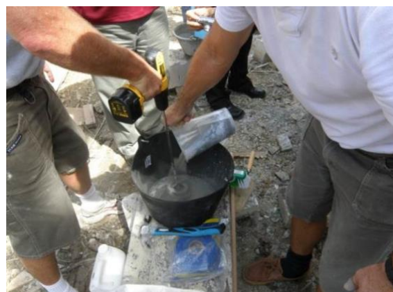
Figure 2 Mixing on site
