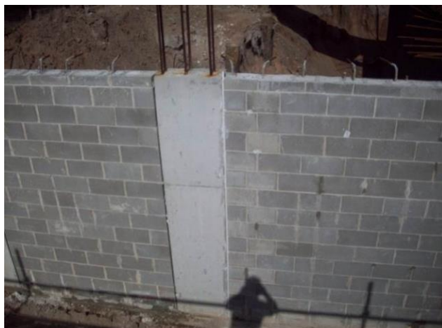
Figure 44 NOVITHOR Flexi-Gel in control joint.
