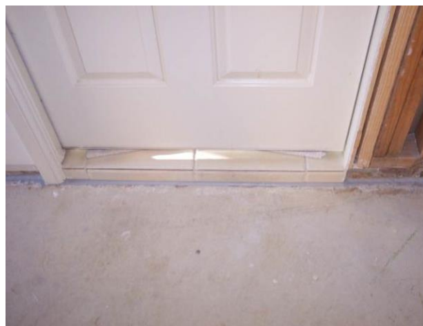
Figure 46 NOVITHOR Flexi-Gel between footing and garage floor in-fill slab.
