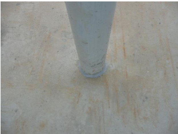
Figure 49 NOVITHOR Flexi-Gel around core drilled pipe.
