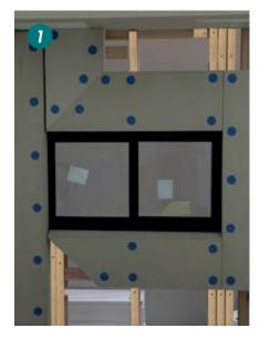
1. Typical window set out with control joint. 8mm gap when forming expansion joint between panels.
