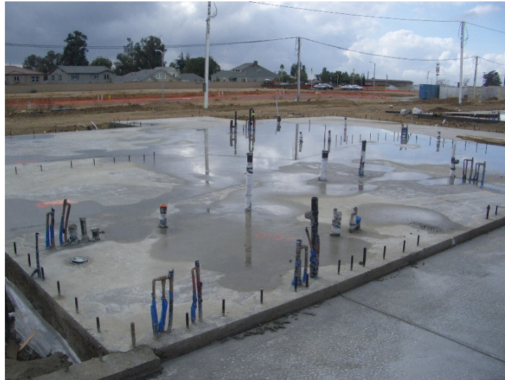
Concrete house slab
