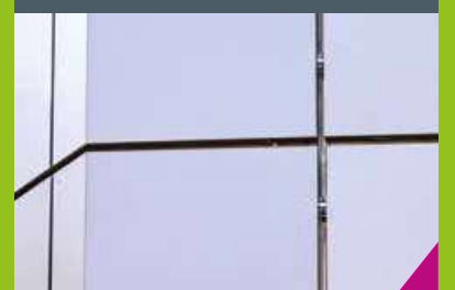
Typical Metal Façade
