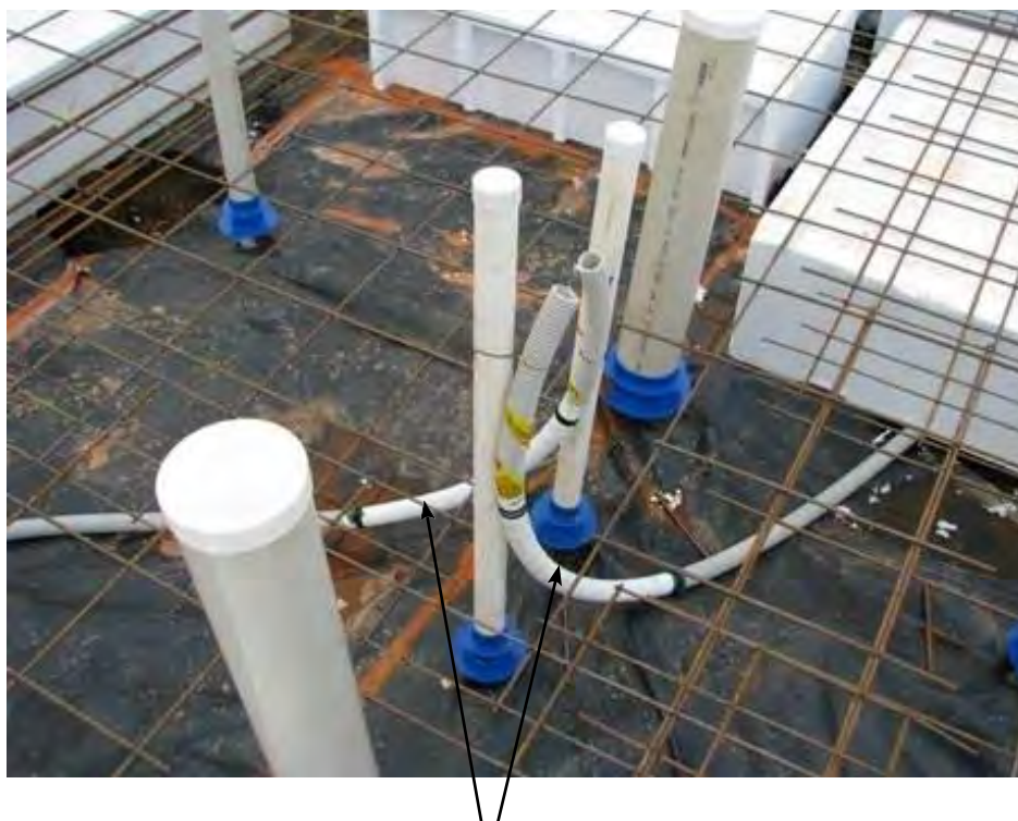
Above image is showing conduit wrapped with HomeGuard® TMB
